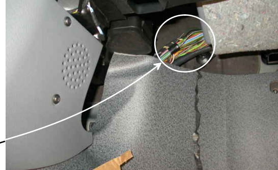
FUSE BOX ENGINE
